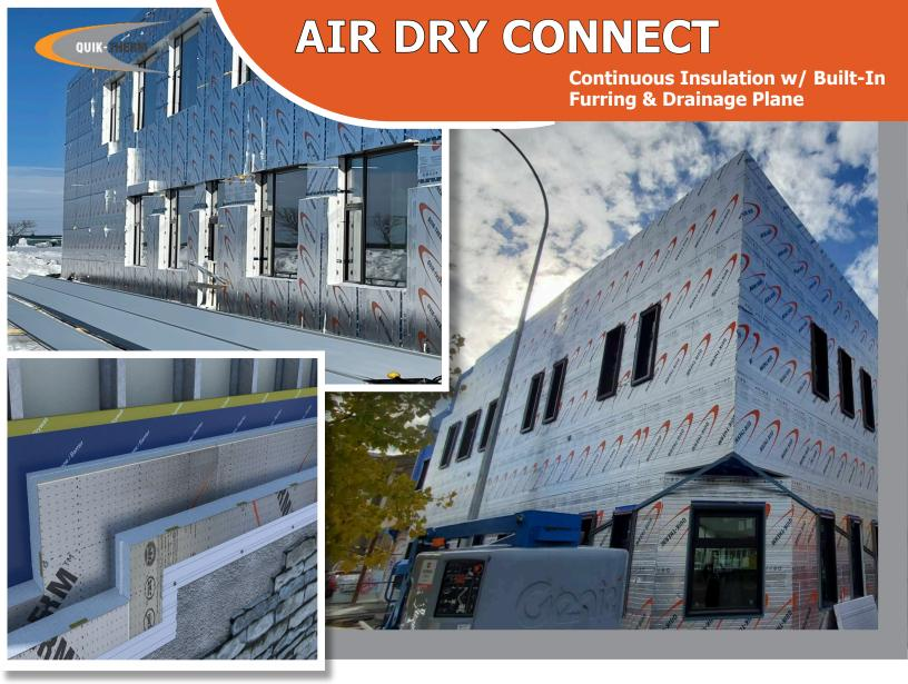
Quik-Therm (QT) Air Dry Connect (ADC) offers a cost-effective, time-saving alternative to traditional rigid insulation and strapping. QT-ADC features a closed-cell expanded polystyrene (EPS) core, with  $\frac{3}{4}$ " thick x 3" wide plywood furring strips embedded into the foam and sealed with perforated reflective polymer facers. The inboard side includes air drainage planes covering 75% of the sheathing surface, reducing hydrostatic pressure and allowing moisture to dry to the exterior.
