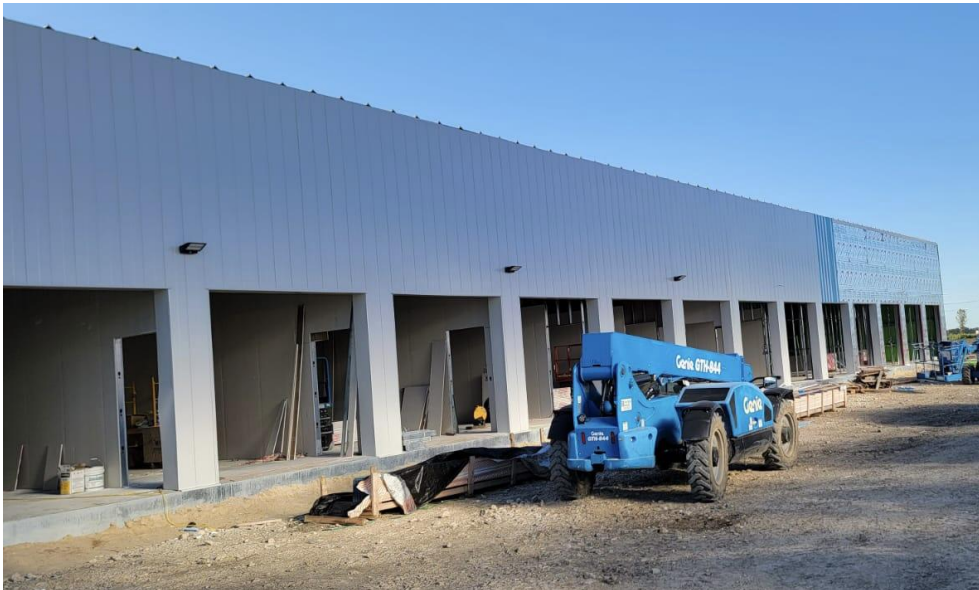
Figure 1. MSG facility in Construction.
