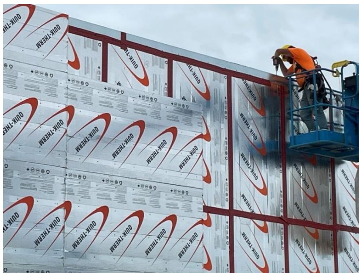
Figure 4. Quik-Therm Matrix System provides a continuous insulation layer, the air barrier, and moisture barrier for the walls and roofs.
