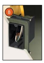
Foam gasket electrical boxes and vapour barrier paint finish the air and vapour control system.
