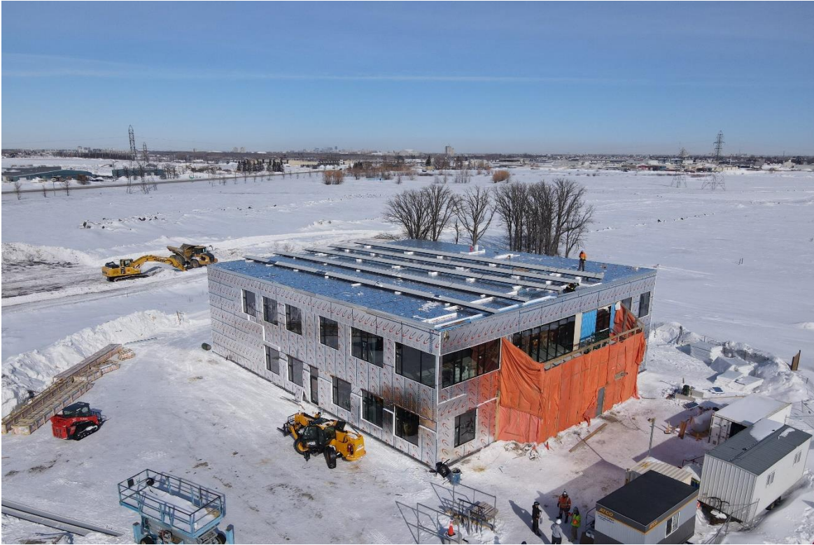
Figure 3. T2K Enterprises HQ Office being insulated with Quik-Therm Exterior Insulation)
