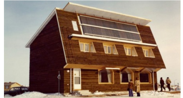
The Conservation House in Saskatchewan was built in 1977, and was a revolutionary building design that introduced passive heating and cooling to modern Passive House construction.
