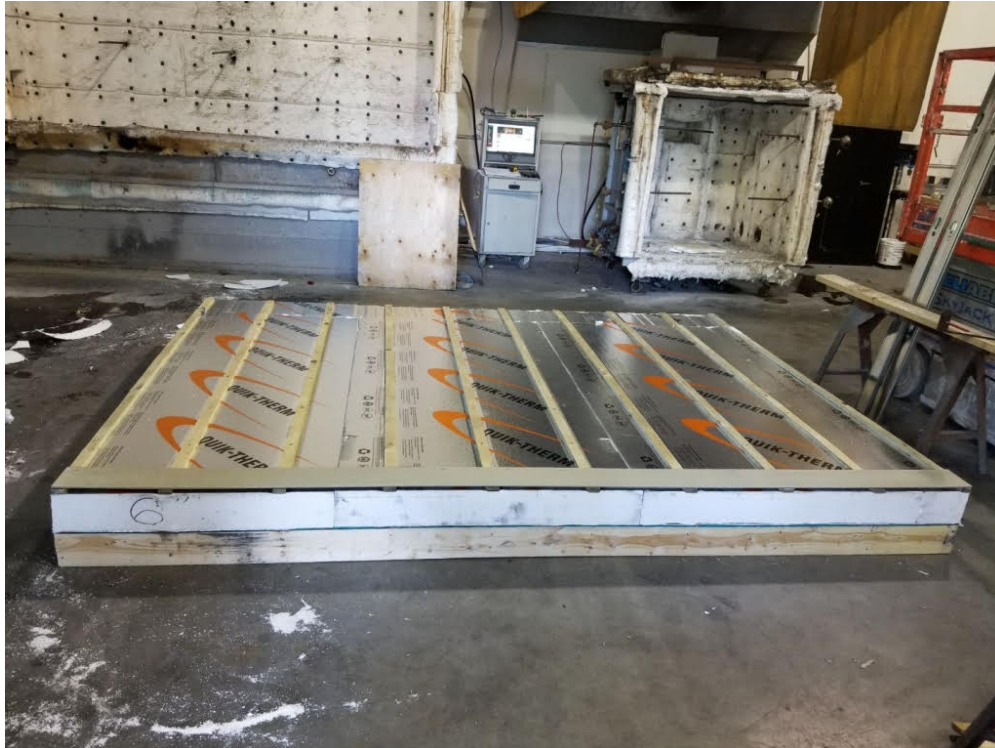
Figure 4: The exposed face prior to installing the cement board lap siding.
