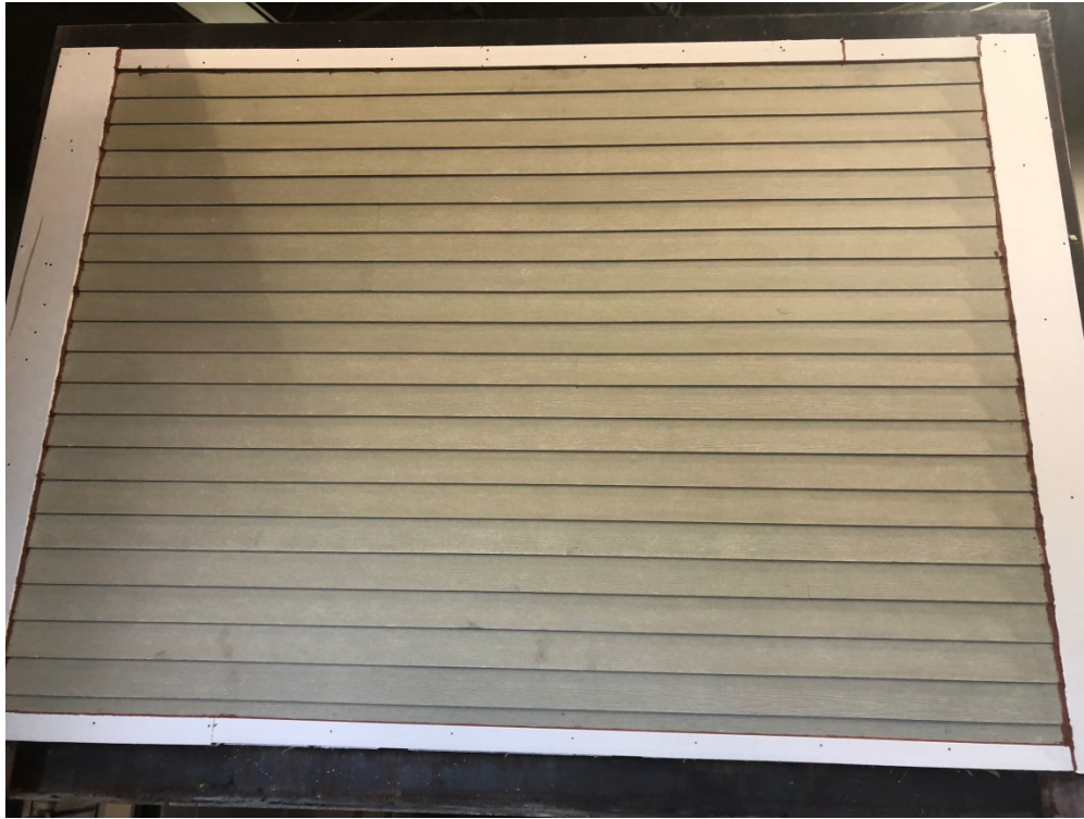
Figure 5: The exposed face prior to the fire test.
