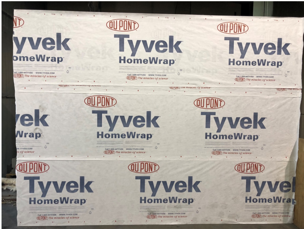
Figure 3: The exposed face prior to installing the Quik-Therm Solar Dry Insulation.
