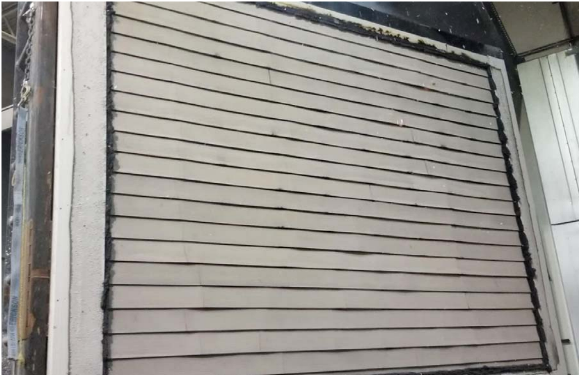
Figure 8: Exposed face after the fire test.
