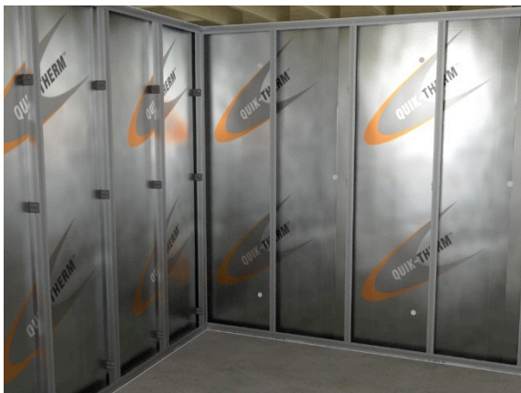
Figure 1: CIS Installed in Basement Application with Steel Framing (L-Studs)
