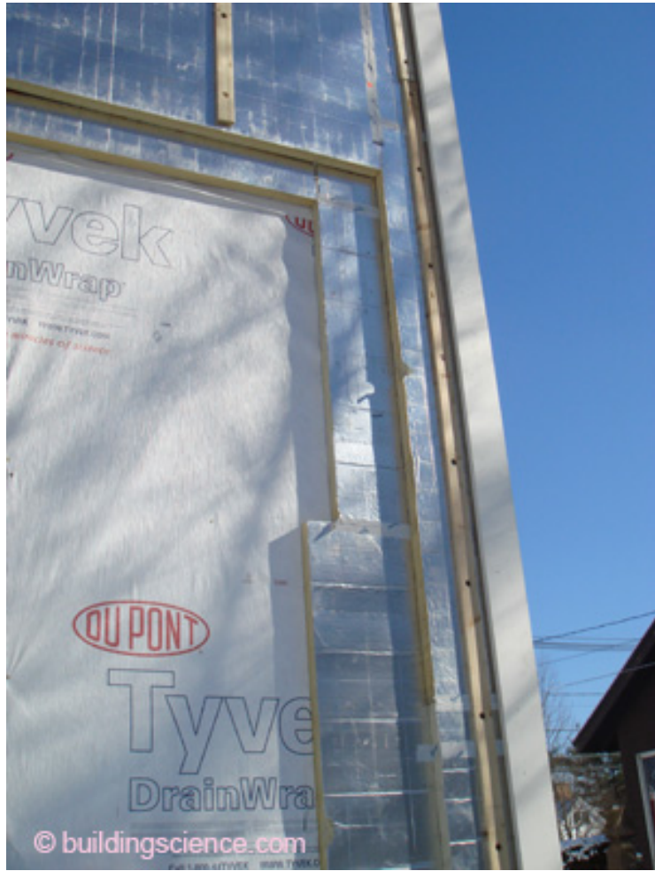
Photograph 11: Perfect Wall Redux —The almost perfect wall has “crinkled” housewrap providing hygric redistribution, 4 inches of foil-faced polyisocyanurate insulating sheathing providing the ultimate thermal break, wood furring providing cladding attachment, relief of hydrostatic pressure and back-ventilation of cladding. OSB under the housewrap provides shear and high-density spray foam cavity insulation (obviously hidden from view) provides air sealing and even more thermal performance. Who says that all these products can’t get along?
