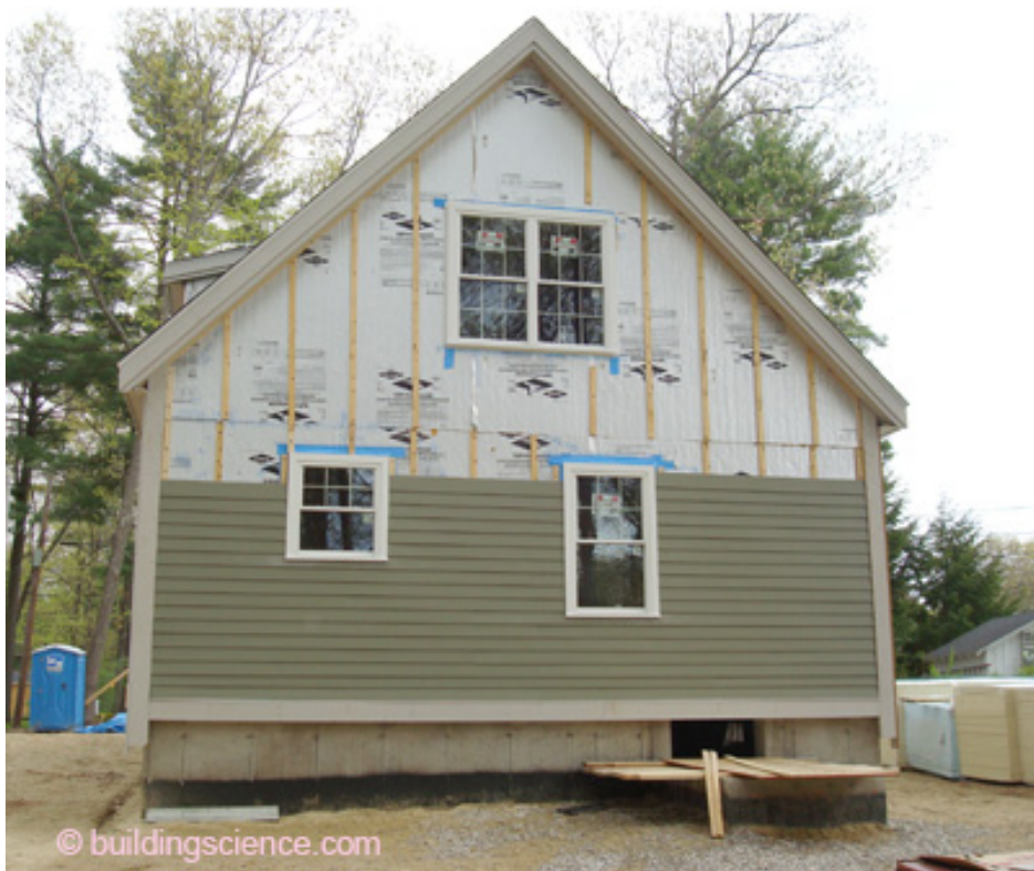
Photograph 7: Furring —When foam sheathings exceed 2 inches in thickness 1x4 furring becomes necessary. This wall has 4 inches of foil-faced polyisocyanurate insulating sheathing installed over a 2x6 wood frame wall. The wood furring acts as the nail base for the fiber-cement cladding.
