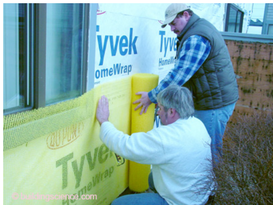
Photograph 3: “High-tech air?” —Polypropylene mesh providing an air gap between OSB covered with housewrap and cladding.
