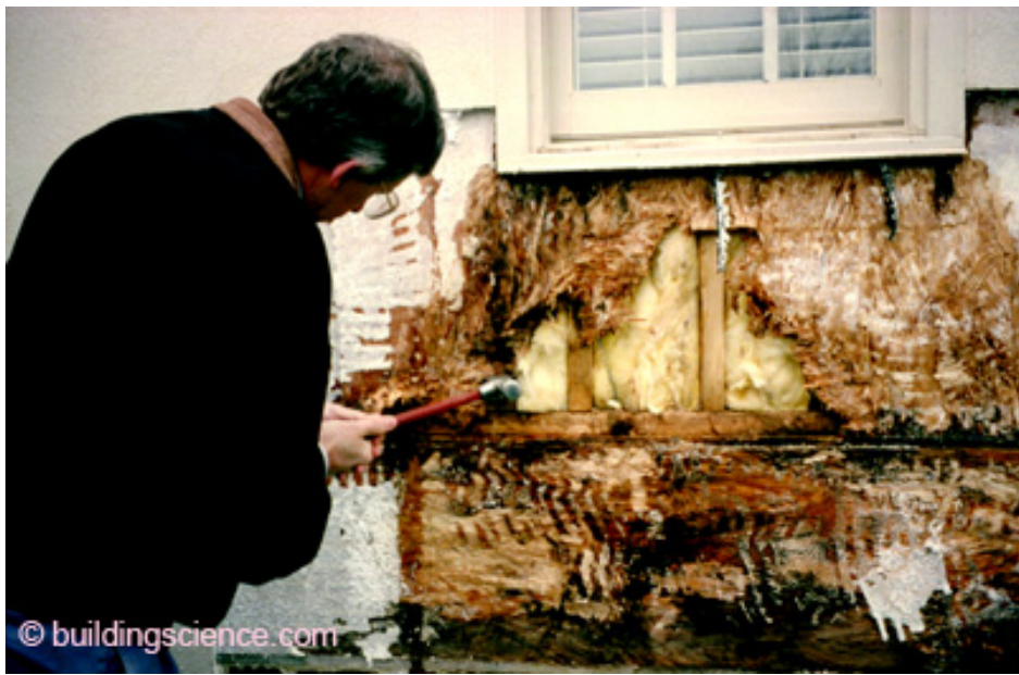
Photograph 8: Nightmare —Exterior Insulated Finish System (EIFS) directly adhered to water sensitive OSB sheathing. Water passes through and around stucco cladding and is trapped between the foam sheathing and the OSB. Water-managed EIFS does not have this problem and is an awesome system.
