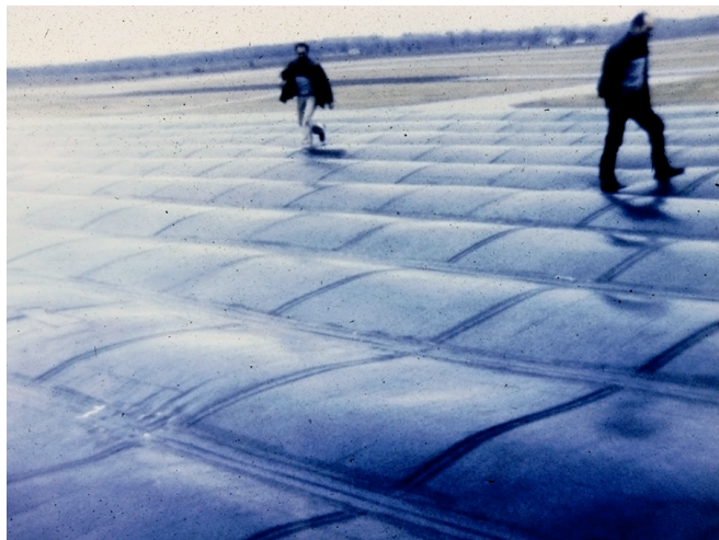
Photograph 1: Missing Air Barrier —With a mechanically attached membrane and no bottom side air barrier the roof membrane “flutters”.
