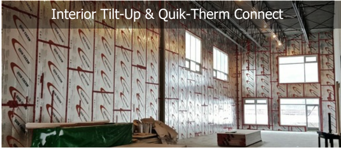
Quik-Therm MPI & Steel Studs
